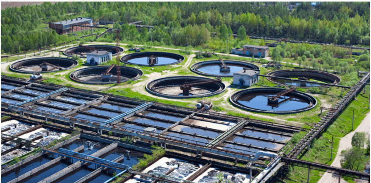
Sewage Treatment Plant ( http://www.boundless.solutions/sewage-treatment-plant/ )
